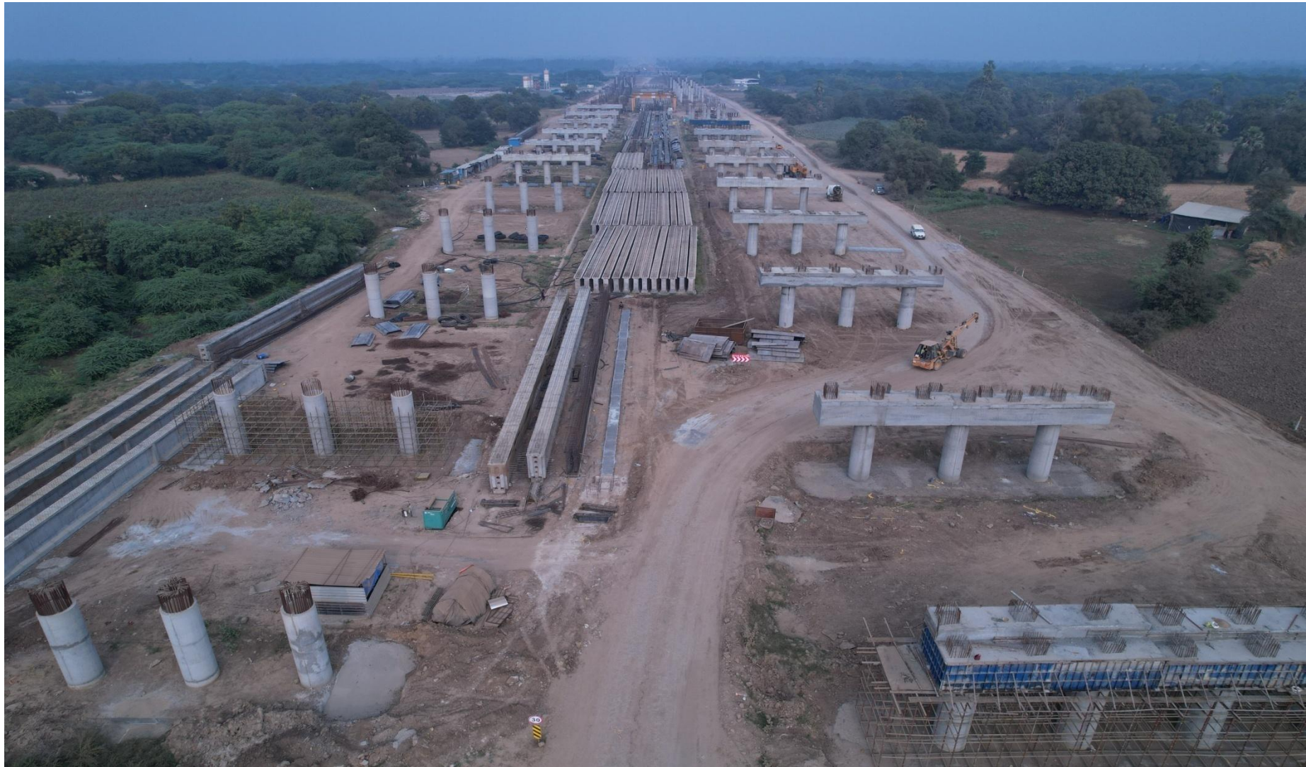
Work In Progress at Major Bridge ch. 352+281 A2 Side
