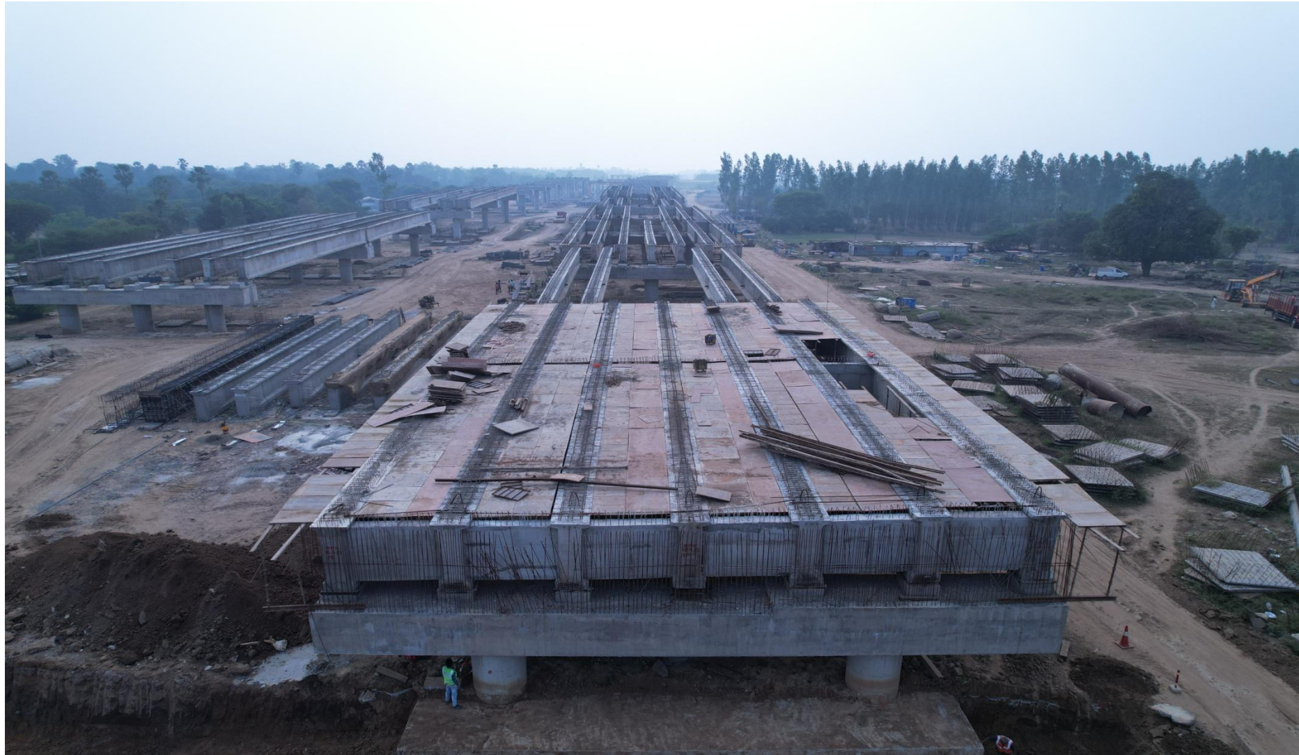
Work In Progress at Major Bridge ch. 352+281 A1 Side
