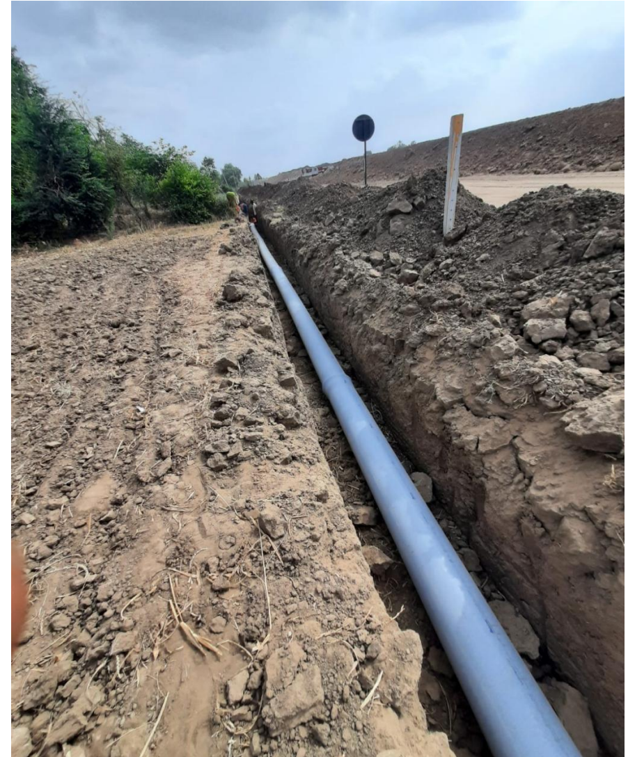
UGPL pipe laying work in progress at Ch. 371+750
