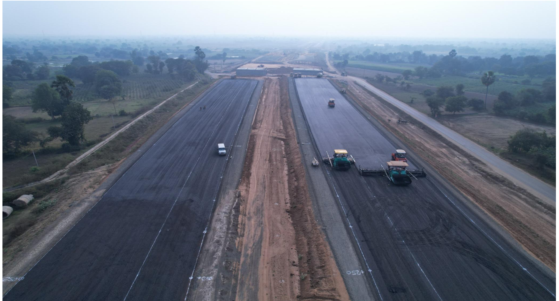
DBM Work In Progress at ch. 359+350
