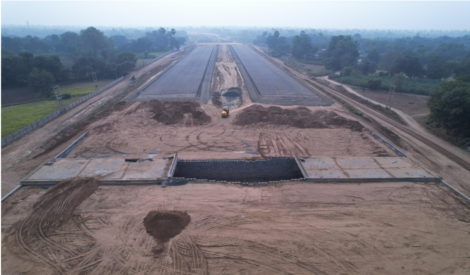
RE - wall Erection work at ch. 354+535 SVUP
