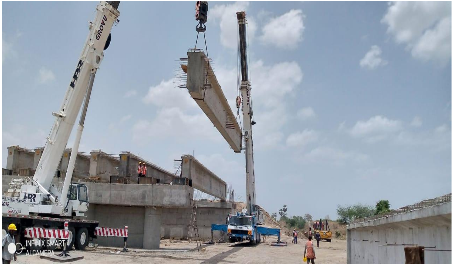
Girder launching at Major Bridge Ch-359+936
