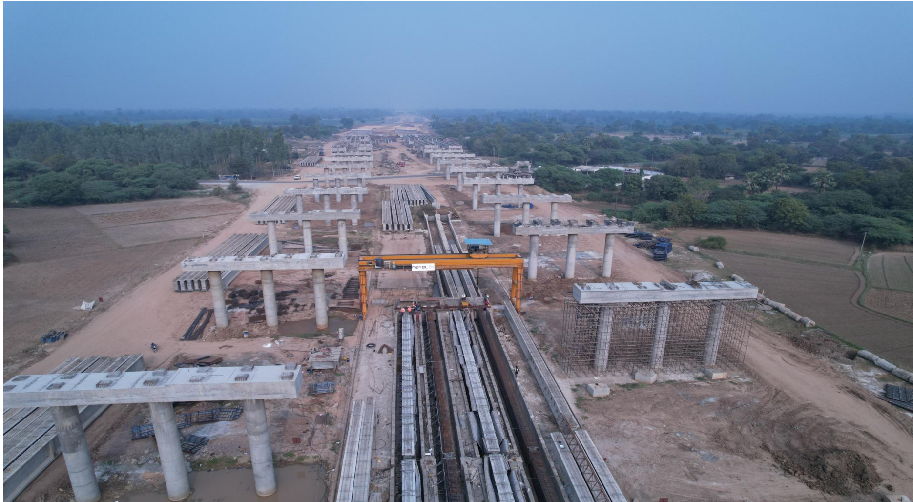
Work In Progress at Major Bridge ch. 352+281 A1 Side
