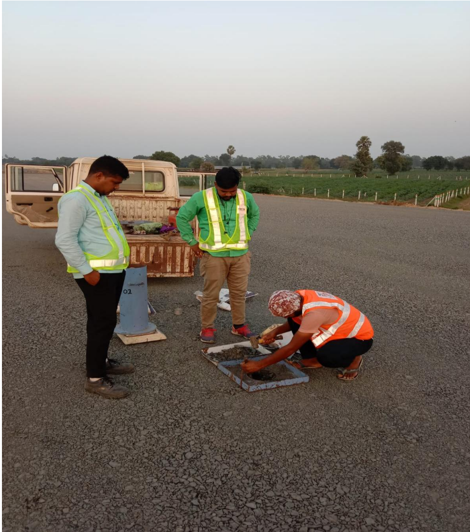
FDD checking at Ch. 351+150 GSB Top
