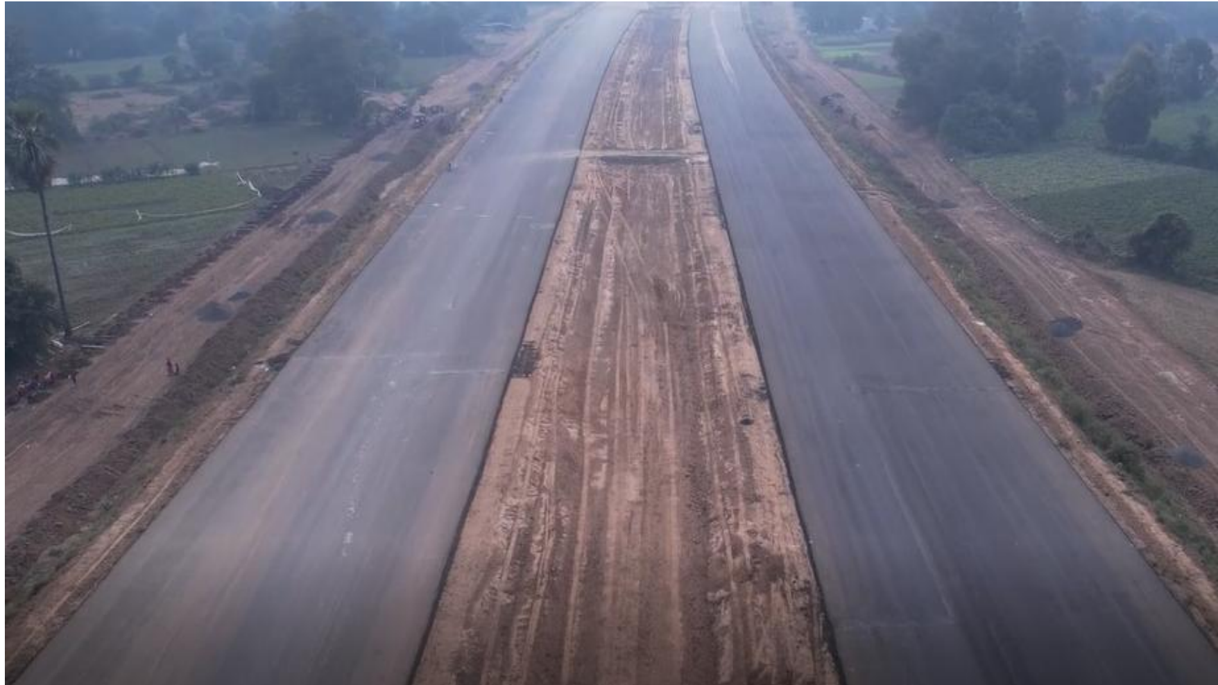
DBM Top Complete at Ch. 353+850
