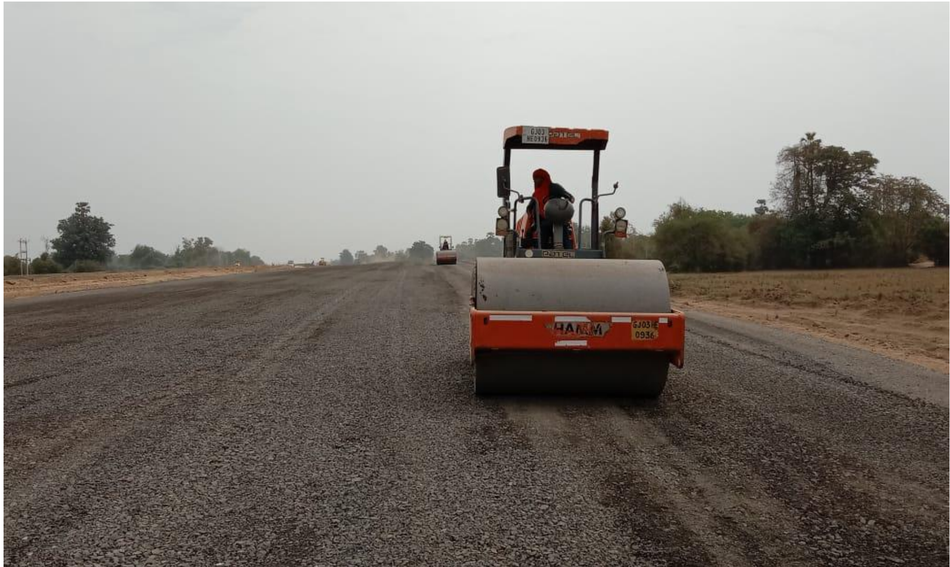
GSB Top Rolling in progress
